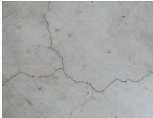
Years of evidence have shown that micro cracks appear in concrete pools for a number of reasons, such as structural ageing, erosion, or ground movements. These small cracks measuring less than 3mm may not affect the structure but can cause a watertightness issue.
